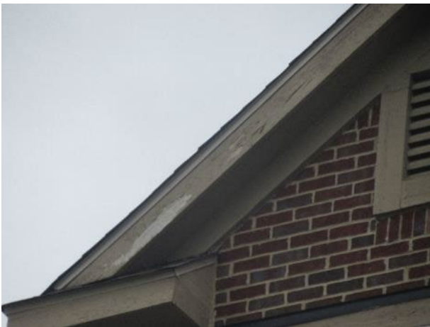
Paint finish deterioration
