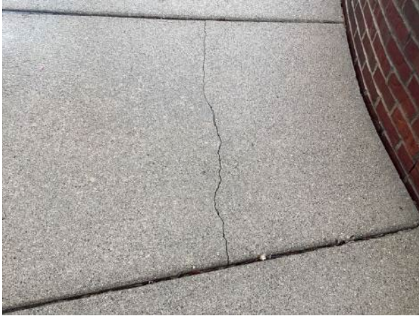
Sidewalk cracks
