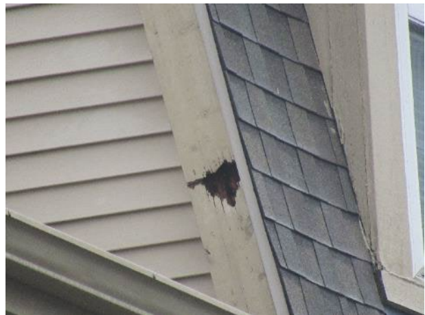
Trim deterioration
