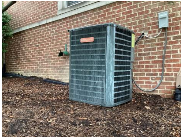
Split system condensing unit
