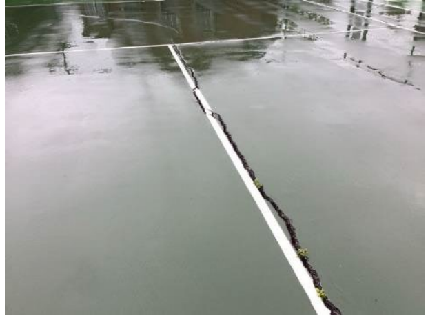
Surface cracks
