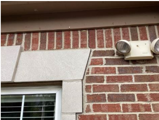
Masonry cracks (clubhouse shown)
