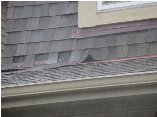
Loose shingles (unit 3047 shown)
