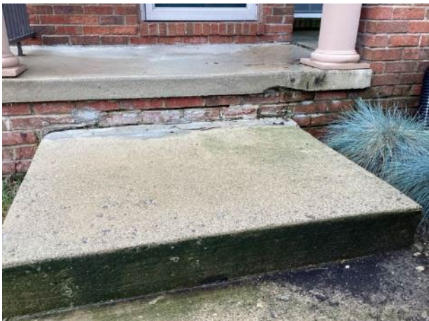
Mortar deterioration and cracks (unit 2798 shown)
