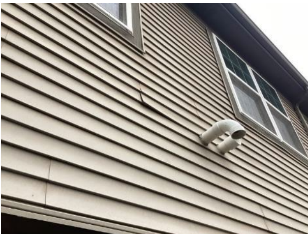
Loose siding (unit 2812 shown)
