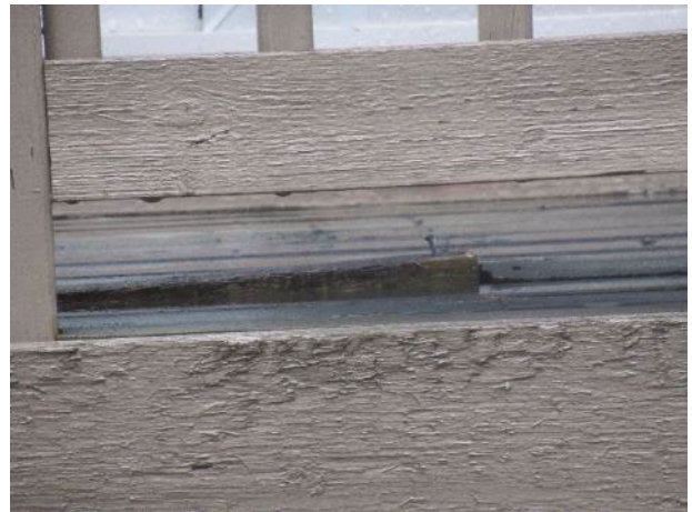
Deck board deflection (unit 2839 shown)
