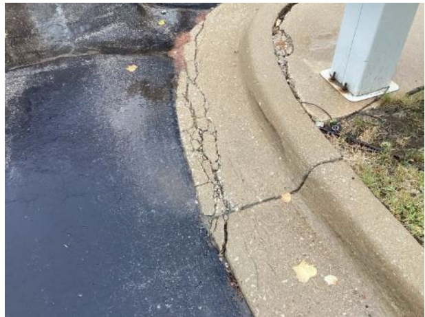
Concrete spalls
