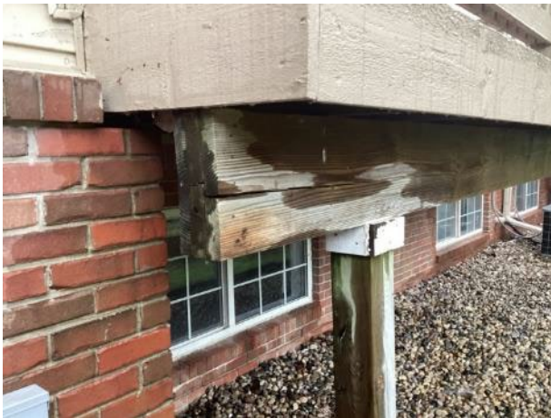
Beam cracks
