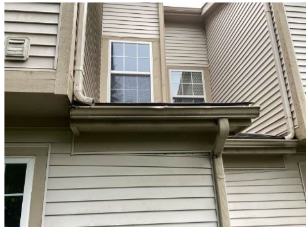
Gutter sloped away from downspout
