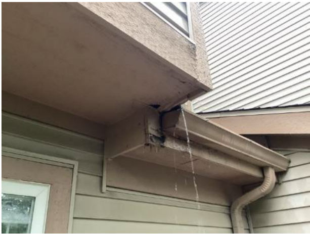
Trim and soffit deterioration
