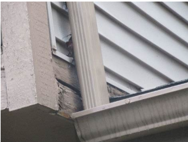
Trim deterioration
