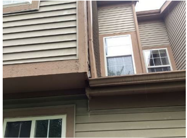
Downspout leakage (unit 2804 shown)
