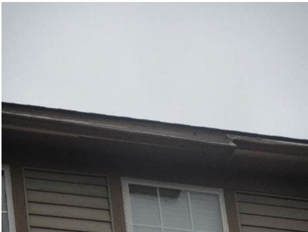
Loose gutter (unit 2792 shown)
