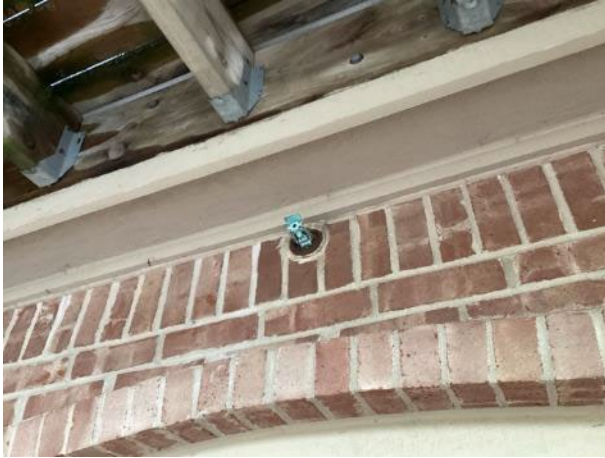
Corroded sprinkler head
