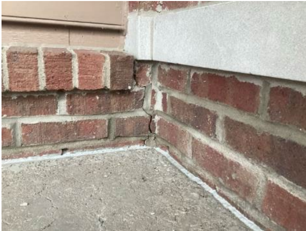
Masonry step cracks (clubhouse shown)
