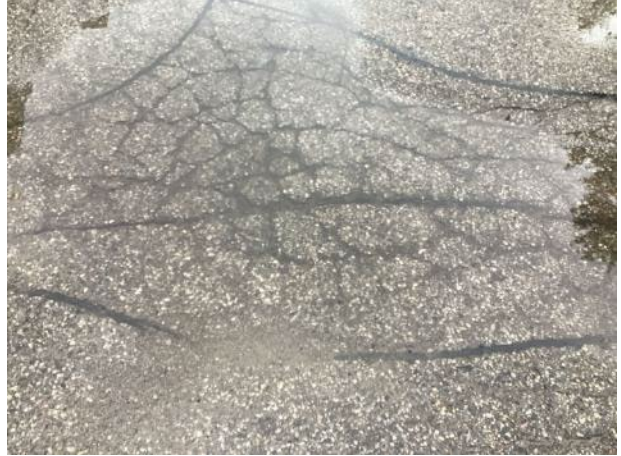
Alligator cracks
