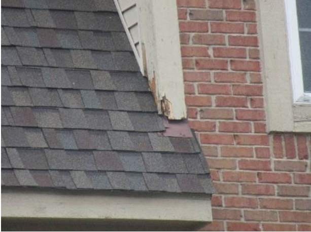
Trim deterioration
