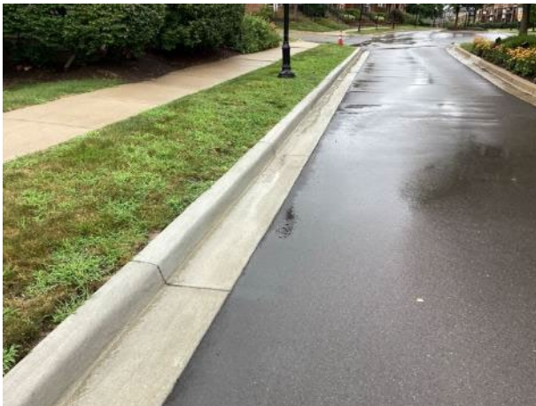
Concrete curb and gutter
