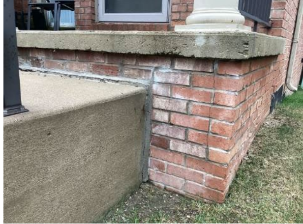
Efflorescence
