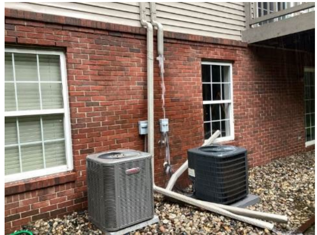
Missing downspout extension (unit 3044 shown)
