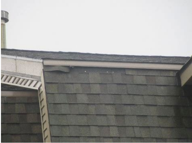
Loose and missing shingles (unit 3030 shown)
