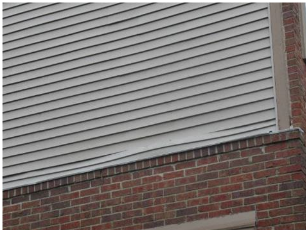
Loose siding (unit 2798 shown)
