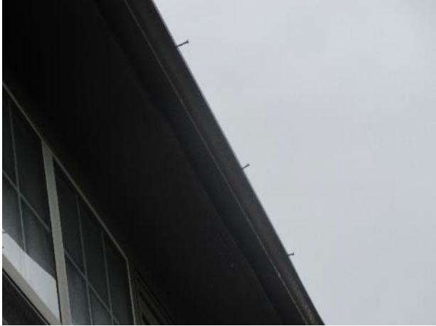
Loose fasteners
