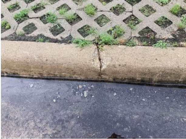
Concrete spalls
