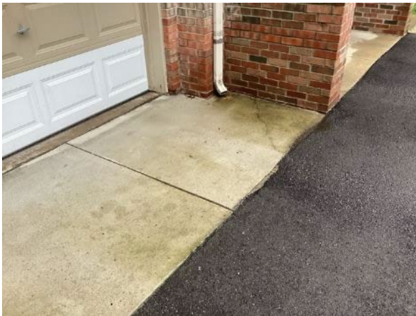
Garage apron cracks
