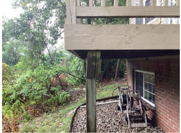
Beam deflection (unit 2958 shown)
