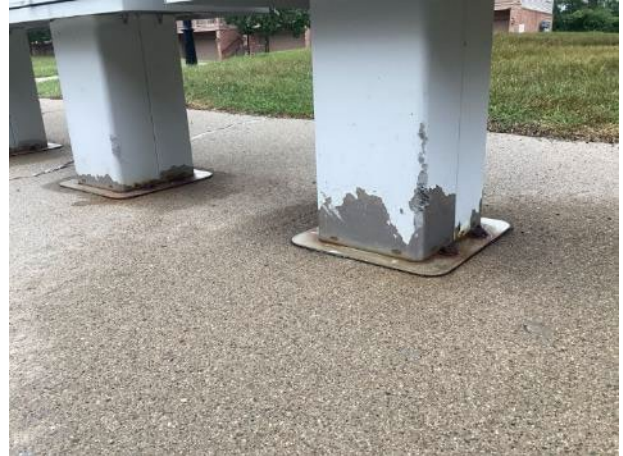
Mailbox station finish deterioration and fastener rust
