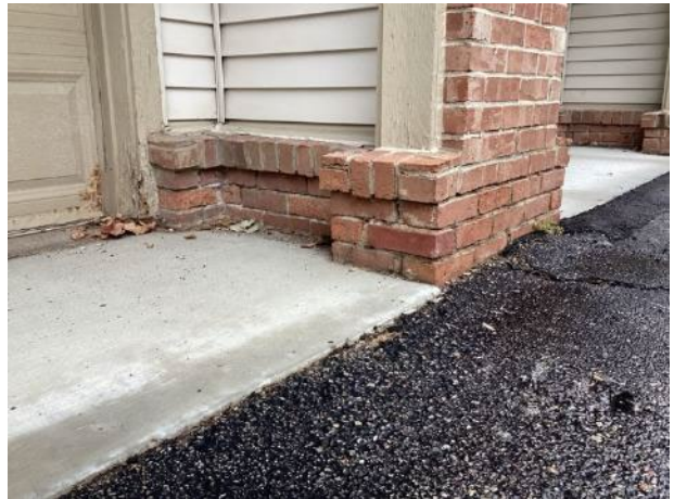
Mortar deterioration and masonry spalls
