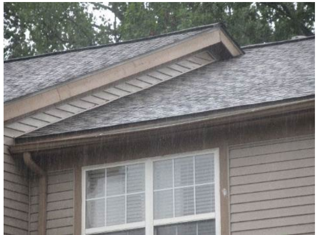
Gutter deflection (unit 2825 shown)
