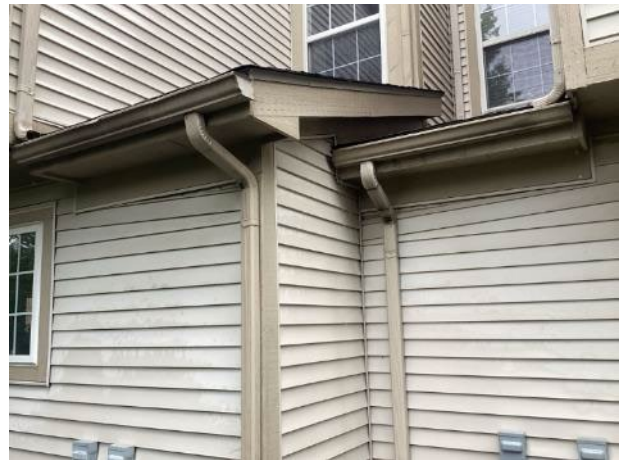
Loose siding (unit 2866 shown)
