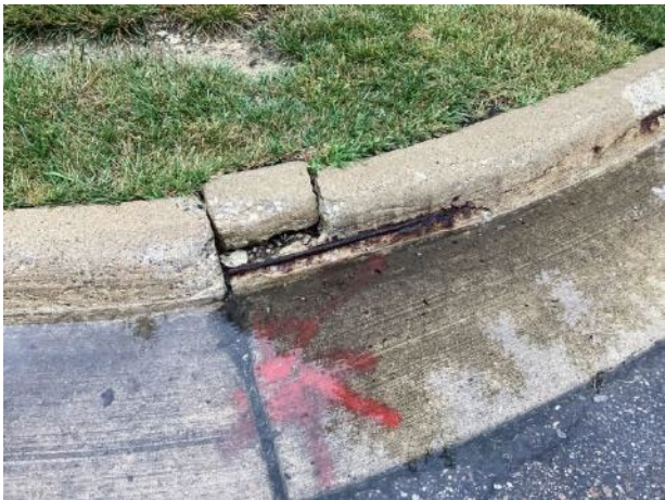
Concrete spalls
