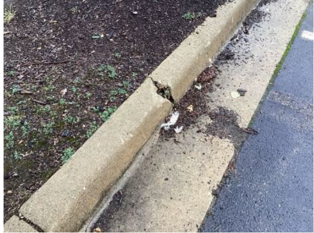
Concrete spalls
