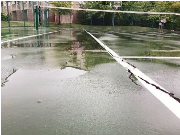
Court settlement and cracks
