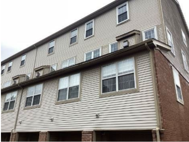
Gutter deflection (unit 2858 shown)
