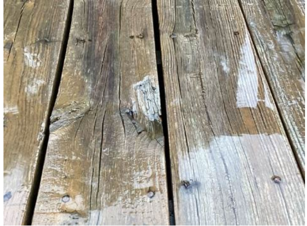
Deck board deterioration
