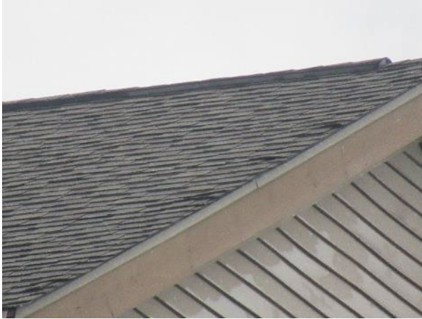
Shingle lift (unit 2865 shown)
