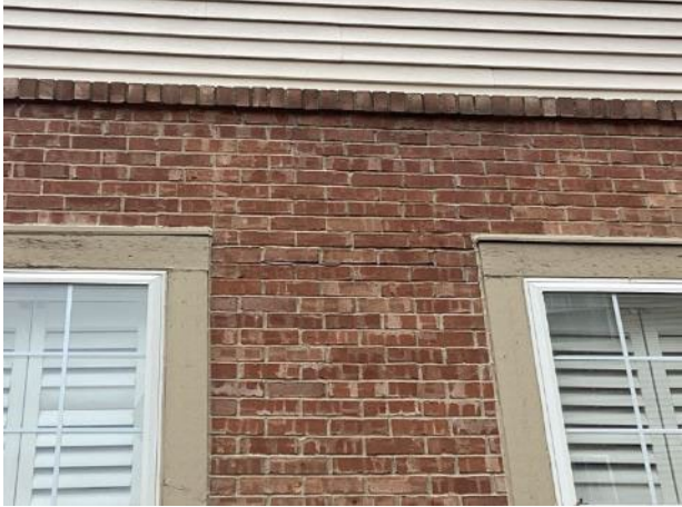
Masonry cracks (unit 2830 shown)
