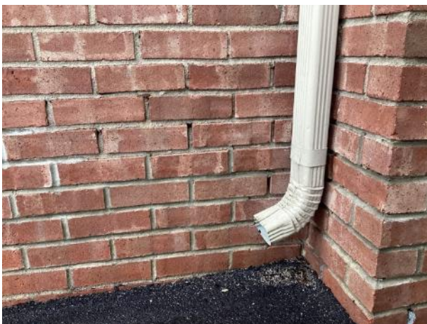
Mortar deterioration
