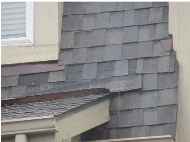
Loose shingles (unit 2767 shown)
