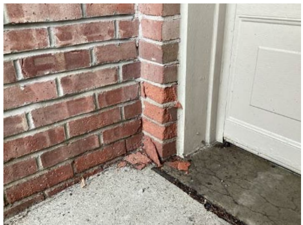
Masonry spall (unit 2768 shown)
