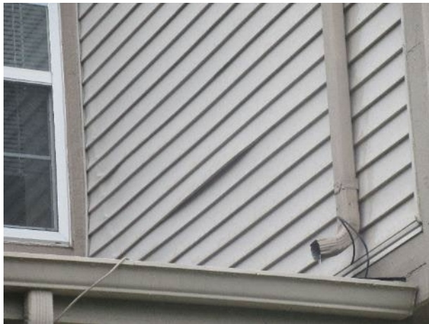
Loose siding (unit 2950 shown)
