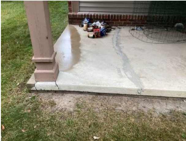
Patio cracks (unit 2804 shown)
