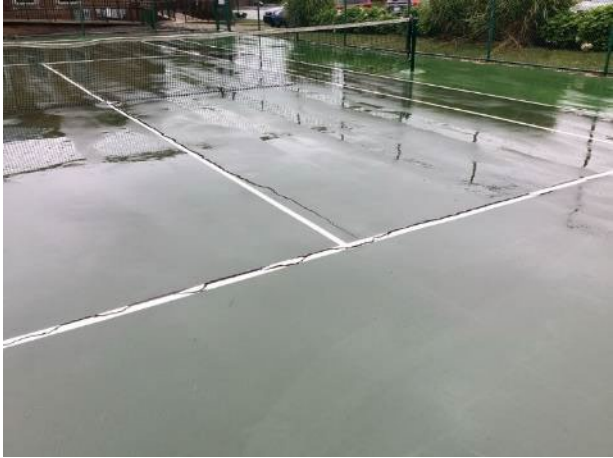
Surface cracks
