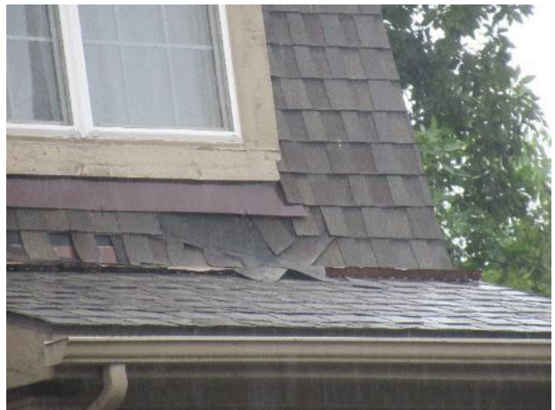
Loose shingles (unit 2723 shown)
