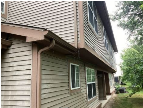
Leakage (unit 2812 shown)
