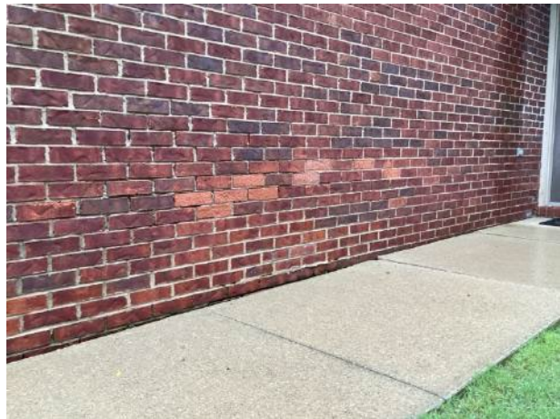
Masonry deterioration (unit 2723 shown)
