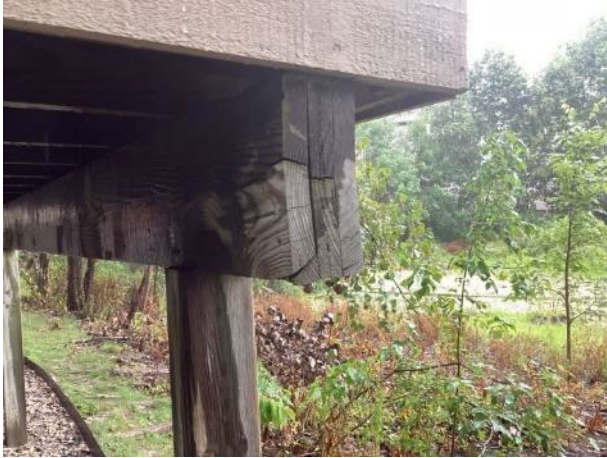
Beam cracks (unit 2968 shown)
