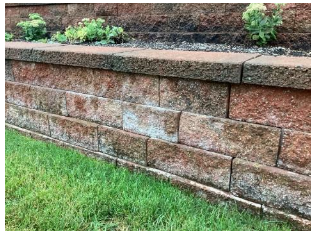
Wall efflorescence
