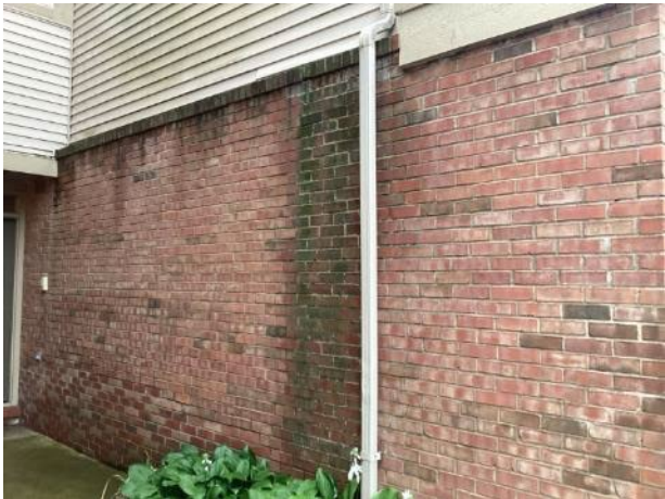
Masonry staining
