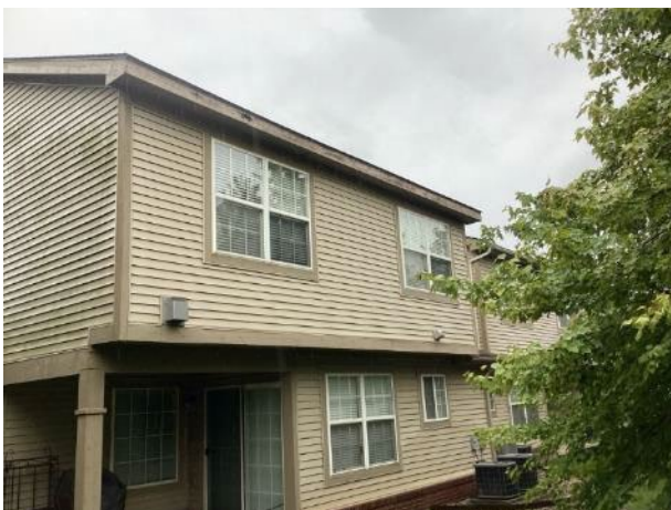
Missing gutter and downspout (unit 2723 shown)
