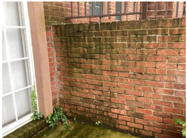
Mortar deterioration
