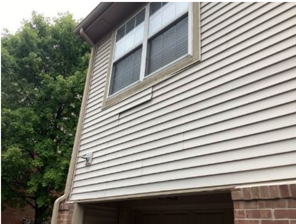
Loose siding (unit 2830 shown)
