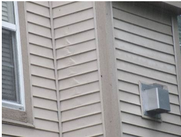
Siding warp (unit 2837 shown)
