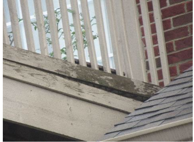
Finish deterioration
