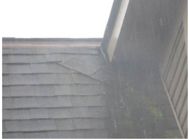
Loose shingles and organic growth (unit 3060 shown)
