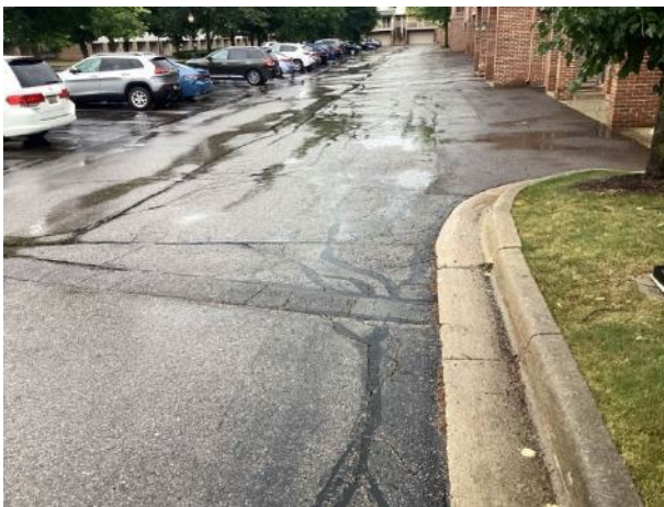
Pavement deterioration
