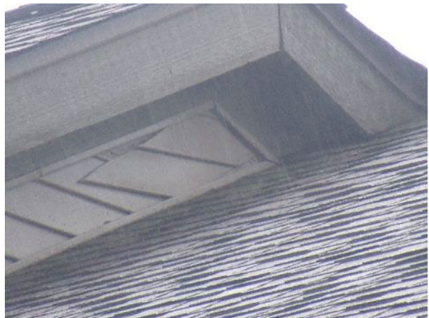
Loose siding (unit 2982 shown)
