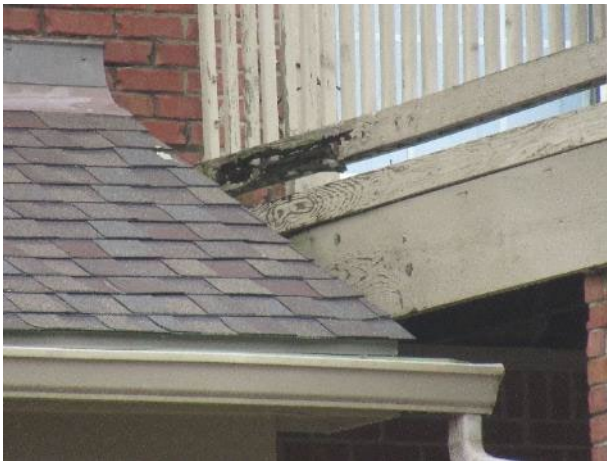
Balcony railing rot (unit 2793 shown)
