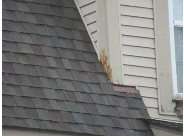
Trim deterioration
