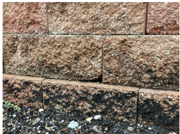
Wall block spall
