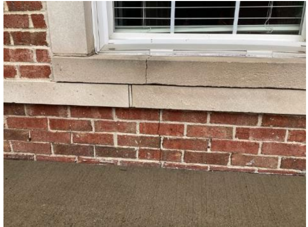
Masonry cracks (clubhouse shown)
