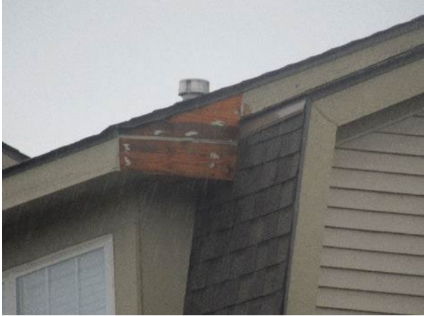
Paint finish deterioration
