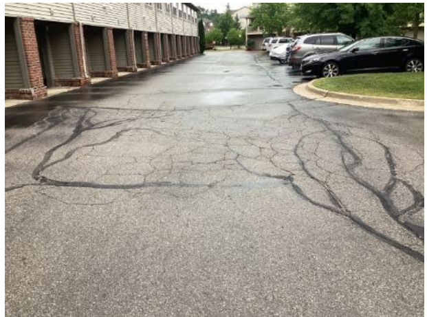
Pavement deterioration
