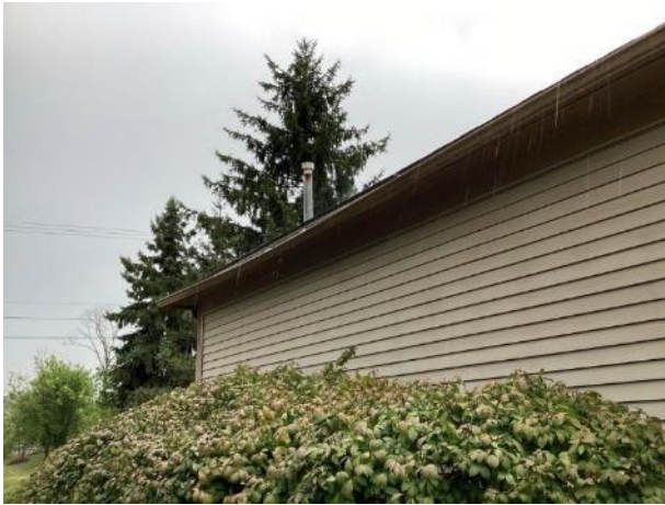
Gutter deflection (garage shown)
