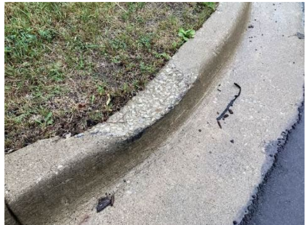
Concrete spalls
