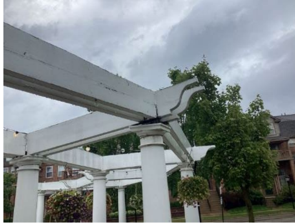
Pergola damage and displacement
