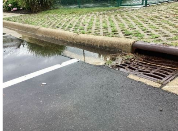
Debris accumulation near catch basin and negative drainage
