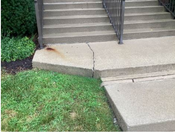
Concrete cracks
