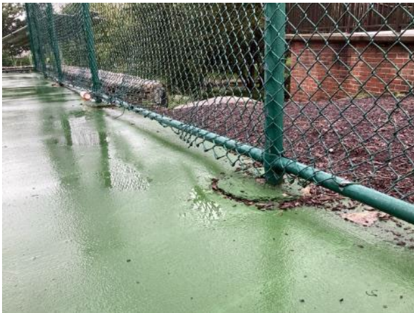
Fence warped webbing
