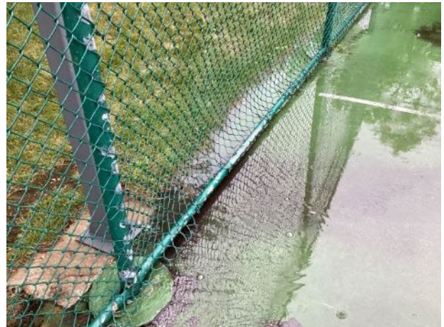
Fence finish deterioration and warped webbing
