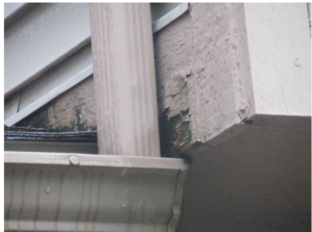
Trim deterioration
