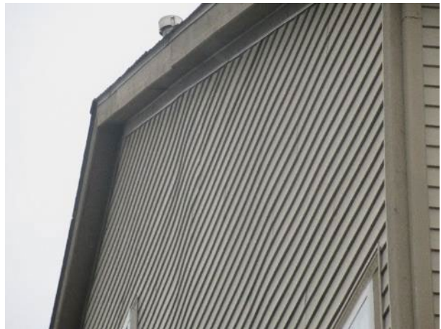
Warped siding (unit 2950 shown)
