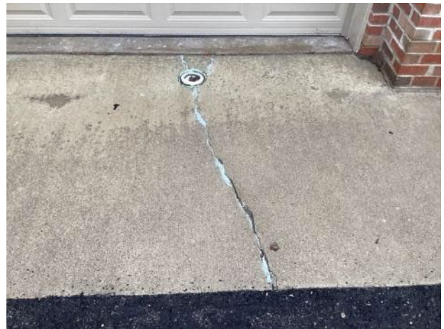
Garage apron cracks
