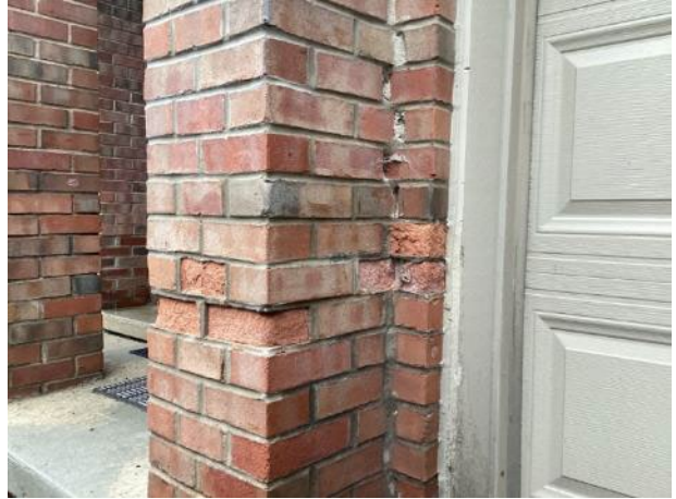
Masonry spalls and mortar deterioration (unit 2874 shown)
